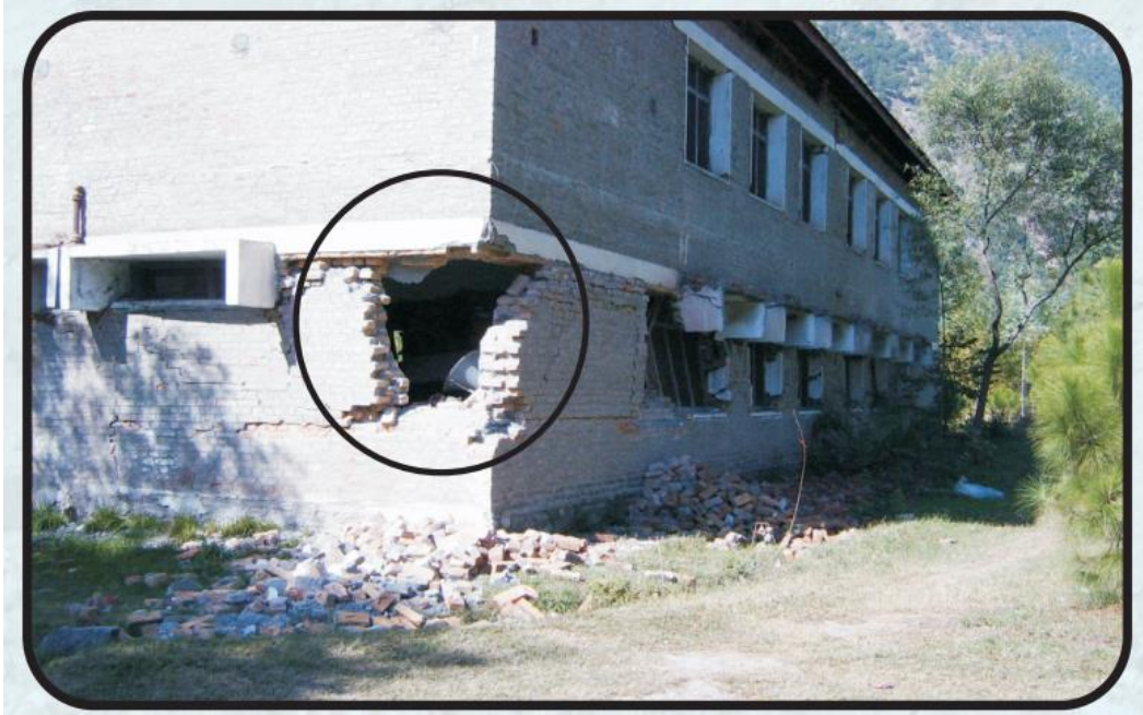
Figure 17-7: Damaged Corner of Building due to Earthquake
